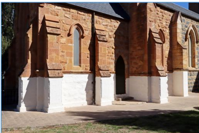
Eroded sandstone on the north face of the chancel, showing damage caused by the past use of non-porous cement mortar.
