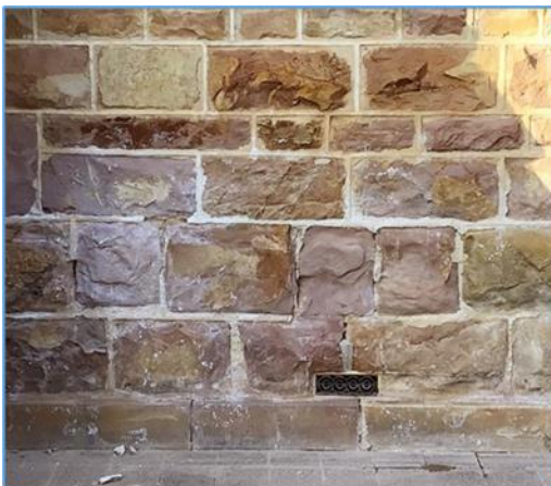
Eroded sandstone on the north face of the chancel, showing damage caused by the past use of non-porous cement mortar.
